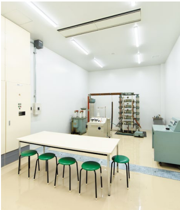
High Voltage Laboratory
